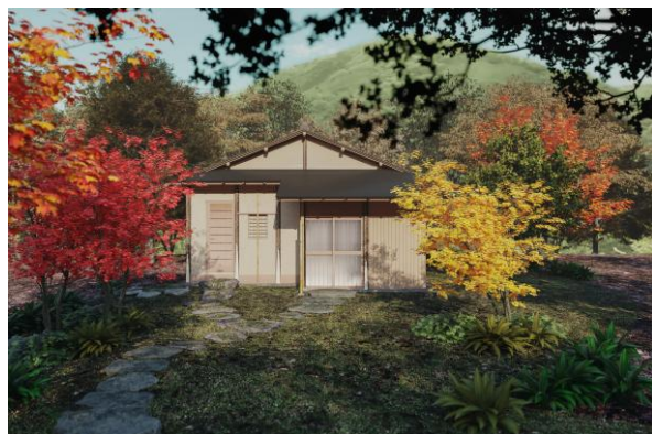
Exterior of the SHIKI-AN
